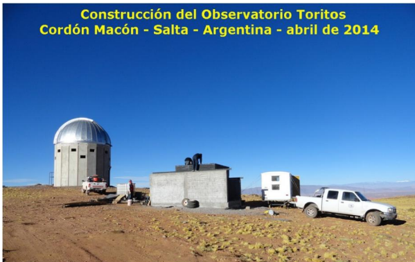
Figure 10: Construction of TOROS at cerro Macón.
